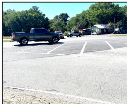
Example of vehicles using the median inconsistently. Vehicle is waiting in the northbound left-turn lane because a vehicle is in the middle of the median.
